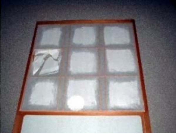
Wet paper to make it easily removed from the door
